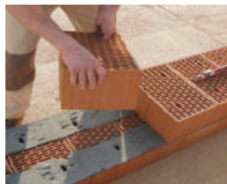
Posa in opera ECOPOR® SSC
