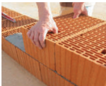
Posa in opera ECOPOR® SSC
